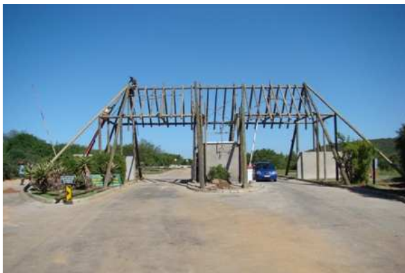
Construction work on the Main Gate
